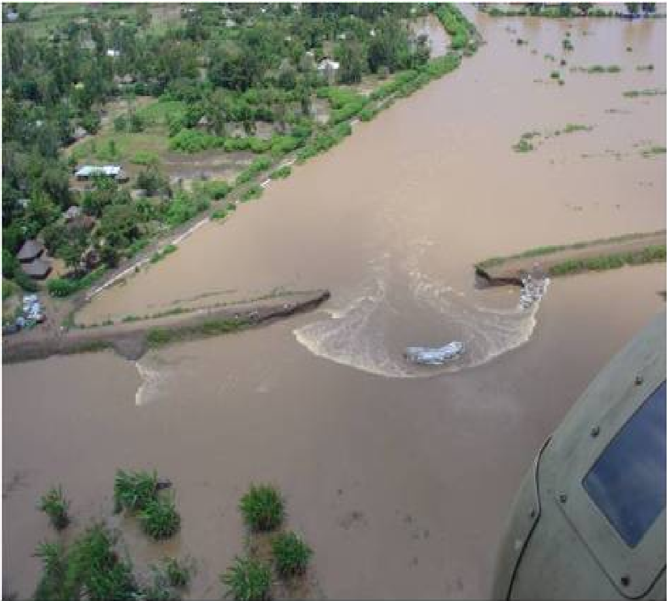
Aerial view of the collapse in the dyke in Budalang'i District
